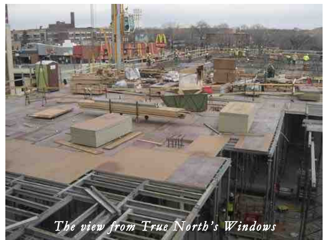
Progress on the Dinkydome and apartments “next door”
